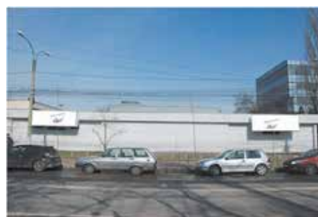
BANNER DISPLAY ON ROMEXPO HEADQUARTER FACADE
